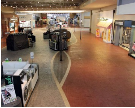
Valley Fair Mall - Renovation Bomanite Thin-Set; Basketweave Used Brick, Random Slate, English Slate Texture, Boardwalk
