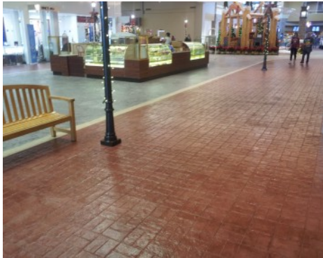
Valley Fair Mall - Renovation Bomanite Thin-Set; Basketweave Used Brick
