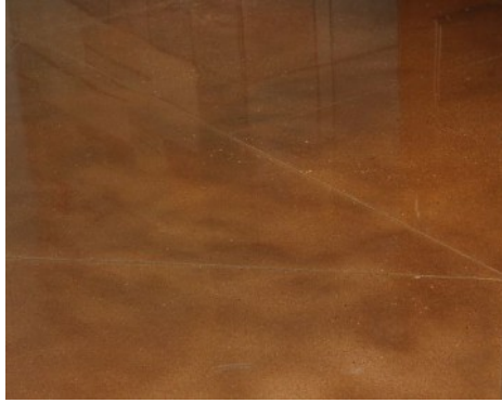
The Summit Recreation Center - Bomanite Integrally Colored Polished Concrete Floor - Close Up
