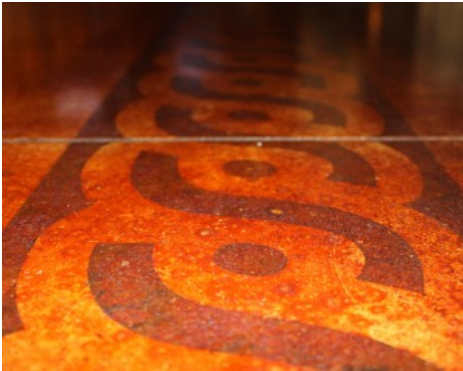
Uncle Julio's Restaurant - Austin Texas Bomanite Chemical Stain and Braided Boarder Stencil
