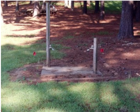
Camp Bud Schiele Cub Scout Rinse Station - Before Installation
