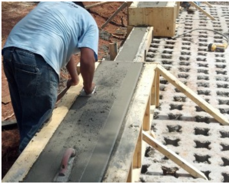
Camp Bud Schiele - Cub Scout Rinse Station - Building Seat Walls
