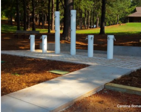
Camp Bud Schiele - Cub Scout Rinse Station - Finished Installation
