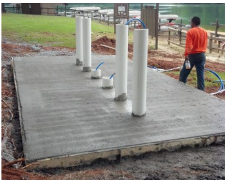
Camp Bud Schiele - Cub Scout Rinse Station - Concrete Pour
