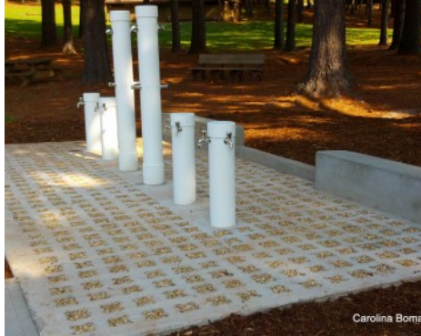
Camp Bud Schiele - Cub Scout Rinse Station - Stone Filled Grasscrete System Finished Installation
