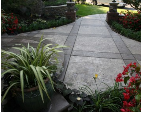
Bomanite Imprinted Concrete - Residential Front Patio - Slate Texture
