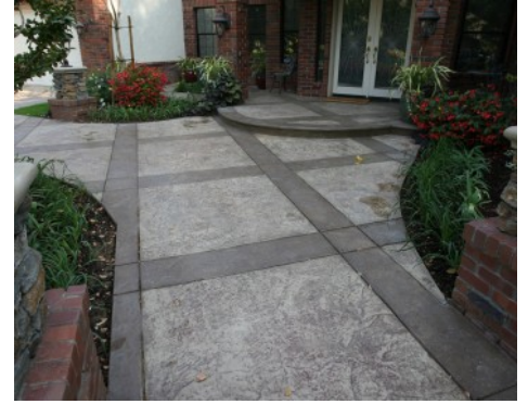
Bomanite Imprinted Concrete - Residential Front Patio - Slate Texture
