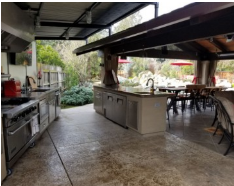
Zuber Residence - Bomanite Exposed Aggregate Systems Antico Process Entertainment Space and Bomanite Imprint System Slate Texture Kitchen
