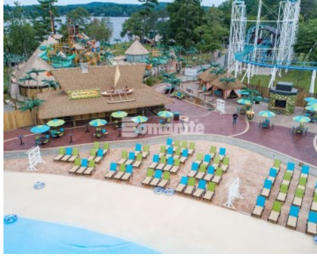
Canobie Lake Park, Castaway Island Expansion by Harrington Bomanite installation of the Walkway and Plaza Stamped with Bomacron 11.5" Boardwalk Pattern and Regular Slate Textured Decorative Concrete
