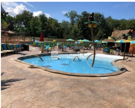
Canobie Lake Park, Castaway Island Expansion by Harrington Bomanite installation of the Kids lagoon Stamped with Bomacron Garden Stone Pattern Decorative Concrete
