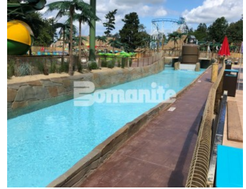
Canobie Lake Park, Castaway Island Expansion by Harrington Bomanite installation of the Tidal River Lifeguard Walk Stamped with Bomacron 11.5" Boardwalk Pattern Decorative Concrete
