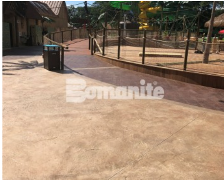
Canobie Lake Park, Castaway Island Expansion by Harrington Bomanite installation of the Walkway and Plaza Stamped with Bomacron 11.5" Boardwalk Pattern and Regular Slate Textured Decorative Concrete
