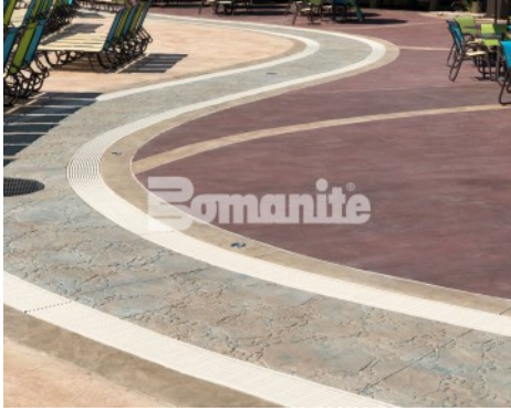
Canobie Lake Park, Castaway Island Expansion by Harrington Bomanite installation of the drainage walkway meandering brook Stamped with Bomacron Garden Stone Pattern Decorative Concrete
