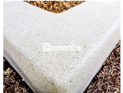
The Coloradan Planter Walls - Bomanite Toppings Systems Micro-Top ST
