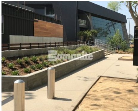
Banc of California LAFC Stadium - Bomanite Exposed Aggregate Systems Sandstone Texture Walkway
