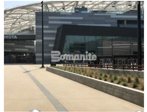
Banc of California LAFC Stadium - Bomanite Exposed Aggregate Systems Sandstone Texture Entry with Bands of Bomanite Alloy
