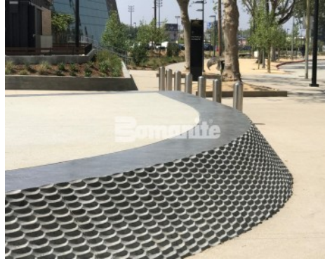
Banc of California LAFC Stadium - Bomanite Exposed Aggregate Systems SandScape Texture Plaza and Flight Wall with Integral Color
