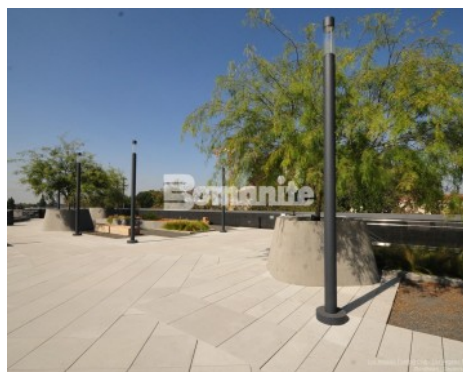
Banc of California LAFC Stadium - Bomanite Exposed Aggregate Systems SandScape Texture Tree Planters and Lineal Planters
