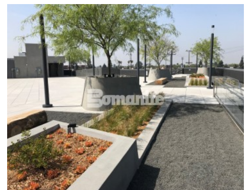
Banc of California LAFC Stadium - Bomanite Exposed Aggregate Systems SandScape Texture Tree Planters and Lineal Planters
