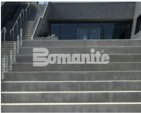
Banc of California LAFC Stadium - Bomanite Exposed Aggregate Systems Sandstone Texture Bench Seats
