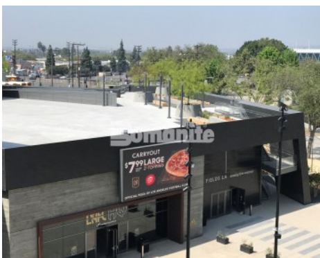
Banc of California LAFC Stadium - Bomanite Exposed Aggregate Systems SandScape Texture Plaza, Roof Top Planters and Bomanite Imprint Systems Boardwalk to Restaurant
