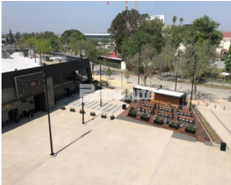
Banc of California LAFC Stadium - Bomanite Exposed Aggregate Systems SandScape Texture Plaza and Bomanite Imprint Systems Boardwalk to Restaurant
