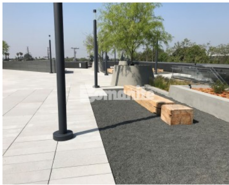
Banc of California LAFC Stadium - Bomanite Exposed Aggregate Systems Sandstone Texture Tree Planters and Lineal Planters
