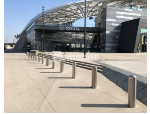
Banc of California LAFC Stadium - Bomanite Exposed Aggregate Systems SandScape Texture Entry with Bands of Bomanite Alloy
