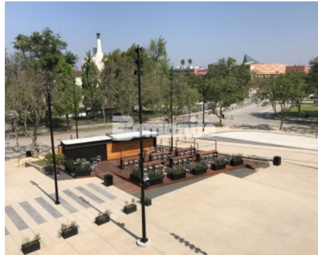
Banc of California LAFC Stadium - Bomanite Exposed Aggregate Systems SandScape Texture Plaza and Flight Wall with Bomanite Imprint Systems
