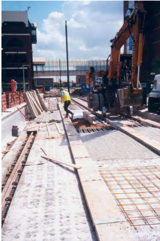
Casting GRASSCRETE slabs with formwork boxes over rail lines
