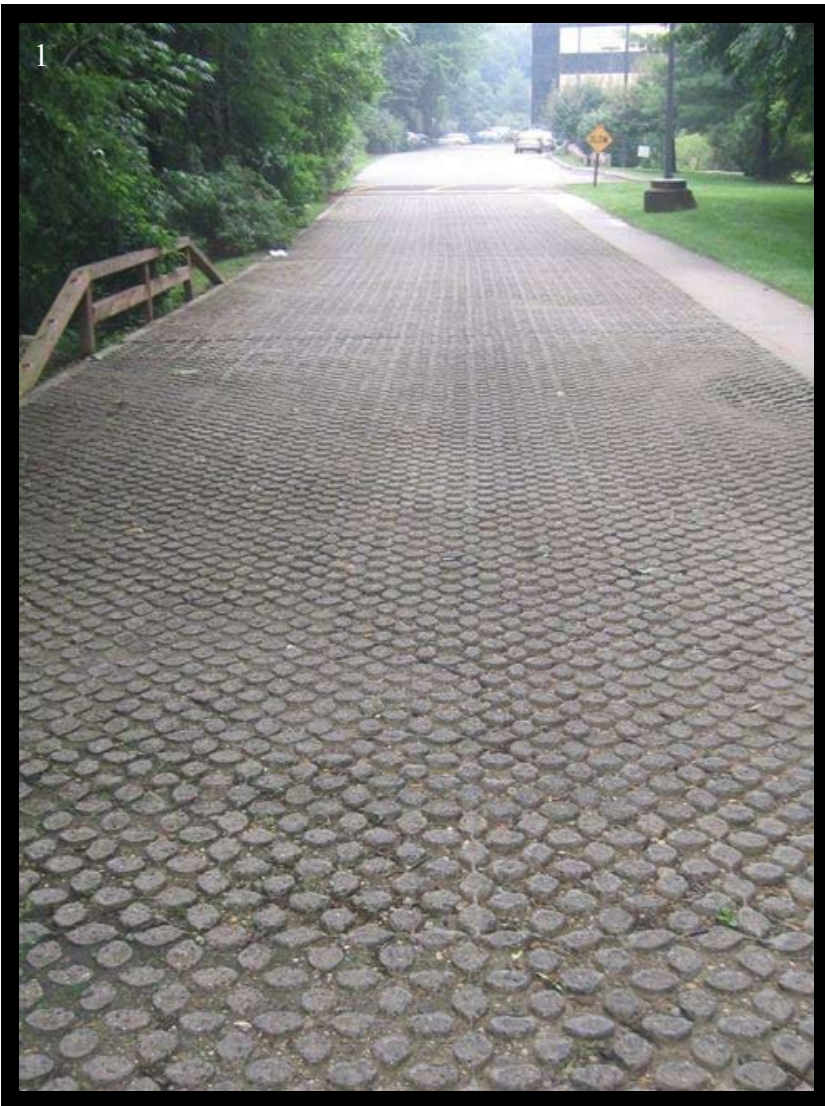
Photo 3: Close-Up of Grasscrete System installed.
