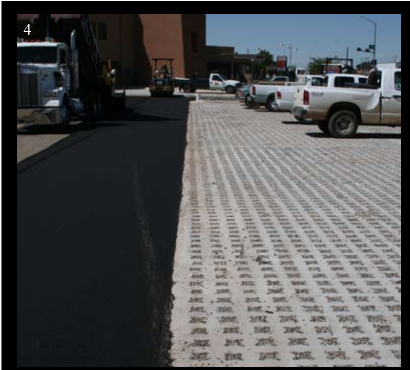
Photo 2: Laying out the Molded Pulp Formers
