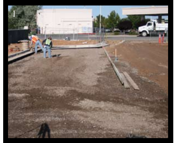
Photo 1: Preparing a base of crushed concrete for the drain bed
