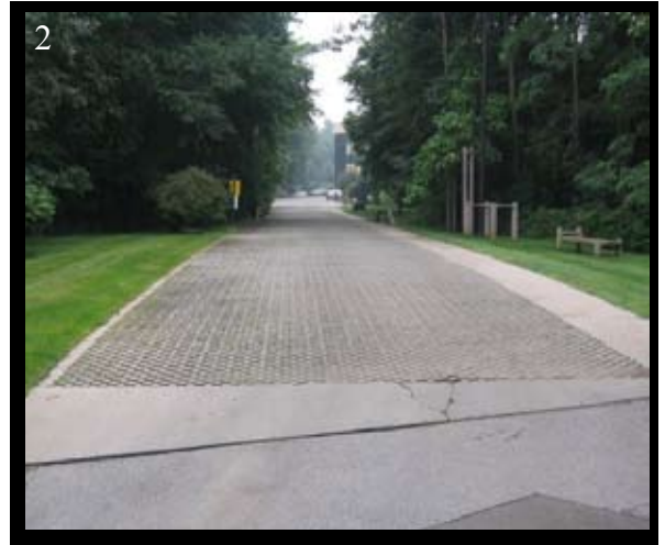
Photo 1: Grasscrete System installed across wetlands to provide access for security and emergency services.
