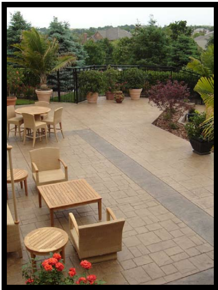
Photo 3: Patio and Deck almost complete
