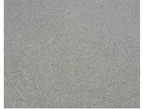
ONE OK Plaza Close Up - Bomanite Alloy
