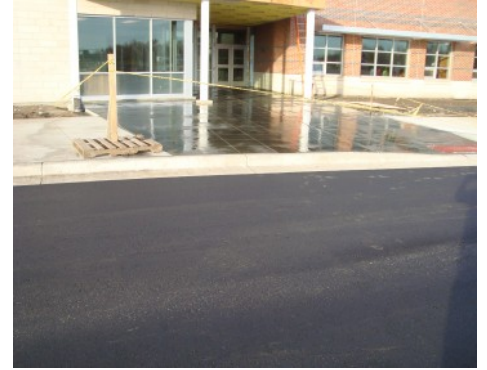
Chapman School Entryway -Installation Bomanite Alloy
