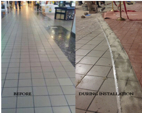
Valley Fair Mall - Before Renovation and during installation
