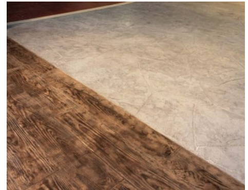
Valley Fair Mall - Renovation Bomanite Thin-Set; Boardwalk, Random Slate,
