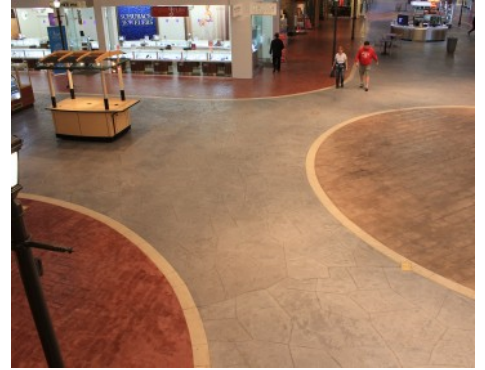
Valley Fair Mall - Renovation Bomanite Thin-Set; Basketweave Used Brick, Random Slate, English Slate Texture, Boardwalk
