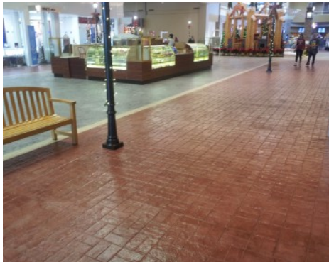
Valley Fair Mall - Renovation Bomanite Thin-Set; Basketweave Used Brick
