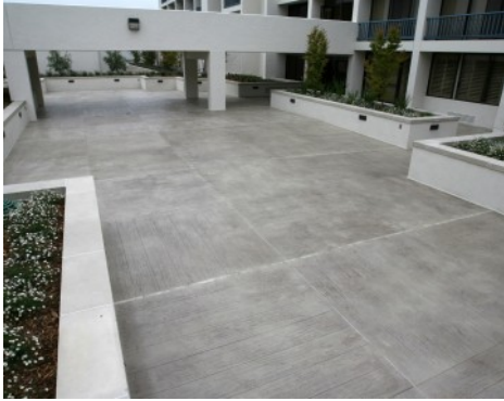
Portola Plaza Hotel - Monterey, CA - Bomanite Thin-Set with Boardwalk Custom Pattern
