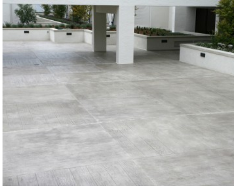
Portola Plaza Hotel - Monterey, CA - Bomanite Thin-Set with Boardwalk Custom Pattern
