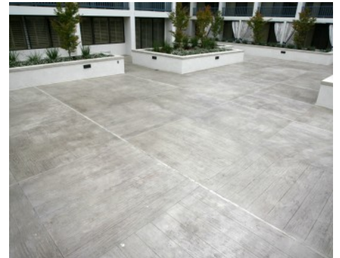
Portola Plaza Hotel - Monterey, CA - Bomanite Thin-Set with Boardwalk Custom Pattern
