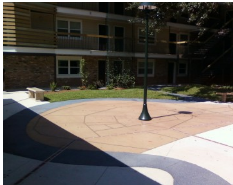
Elysian Courtyard - Bomanite Revealed
