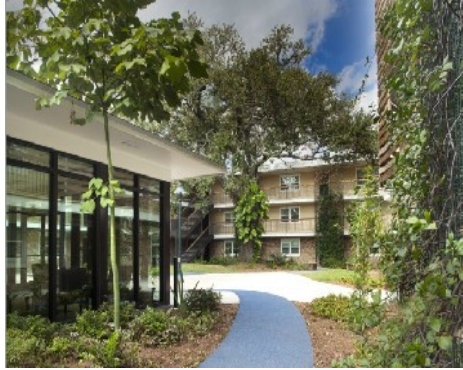
Elysian Courtyard - Bomanite Revealed
