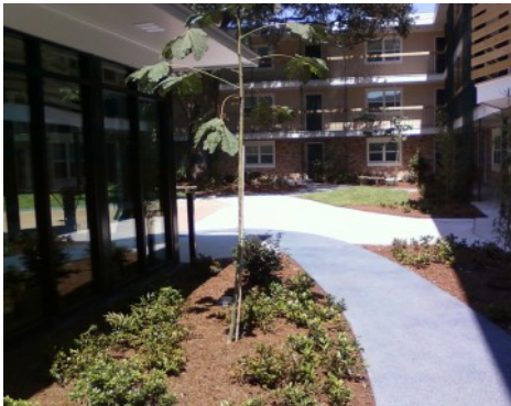
Elysian Courtyard - Bomanite Revealed
