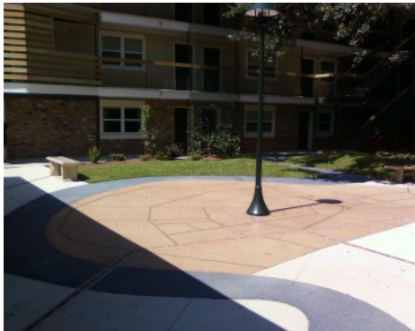
Elysian Courtyard - Bomanite Revealed
