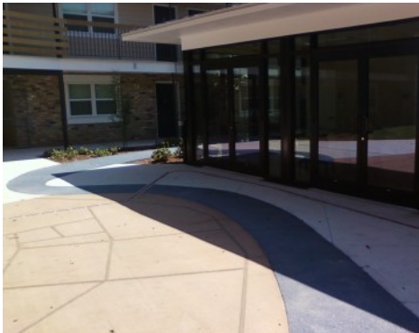
Elysian Courtyard - Bomanite Revealed
