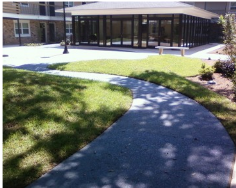
Elysian Courtyard - Bomanite Revealed
