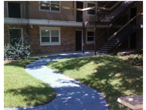
Elysian Courtyard - Bomanite Revealed
