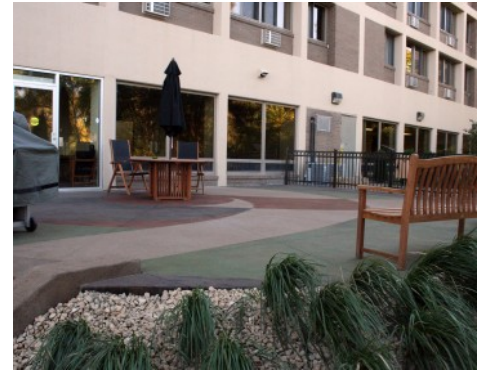
Nan McKay Public Housing - Bomanite Sandstone and Chemical Stain
