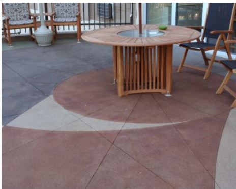
Nan McKay Public Housing - Bomanite Sandstone and Chemical Stain
