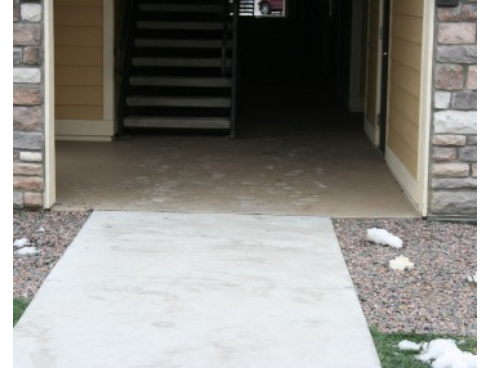
Broadstone Apartments - Bomanite Broadcast Aggregate System
