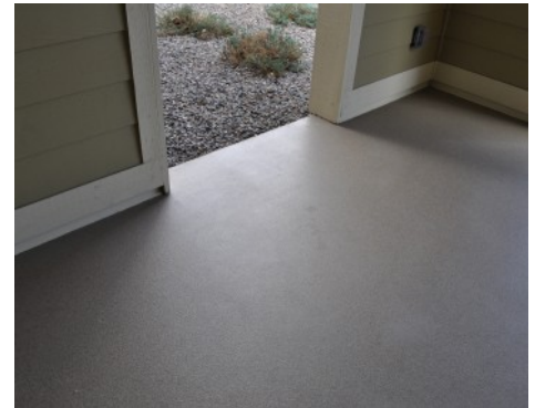
Broadstone Apartments - Bomanite Broadcast Aggregate System
