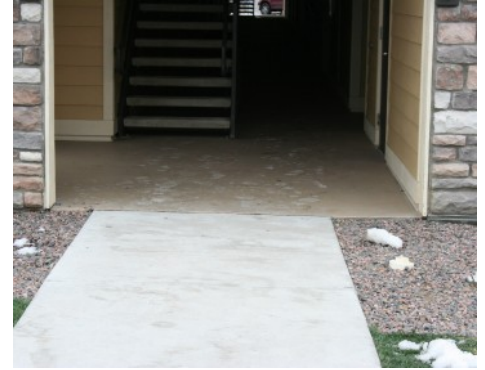
Broadstone Apartments - Bomanite Broadcast Aggregate System
