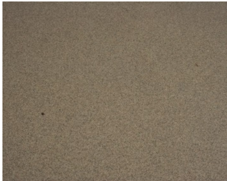
Broadstone Apartments - Bomanite Broadcast Aggregate System
