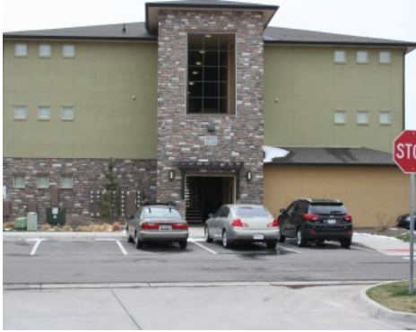
Broadstone Apartments - Bomanite Broadcast Aggregate System
