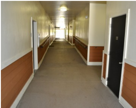
Broadstone Apartments - Bomanite Broadcast Aggregate System
