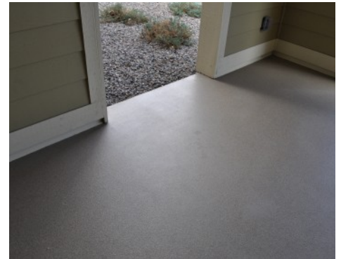
Broadstone Apartments - Bomanite Broadcast Aggregate System
