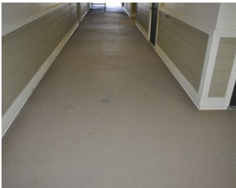
Broadstone Apartments - Bomanite Broadcast Aggregate System
