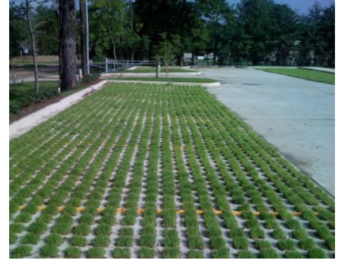
LA Army National Guard - Grasscrete Parking Lot
