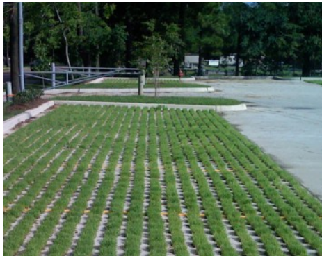
LA Army National Guard - Grasscrete Parking Lot
