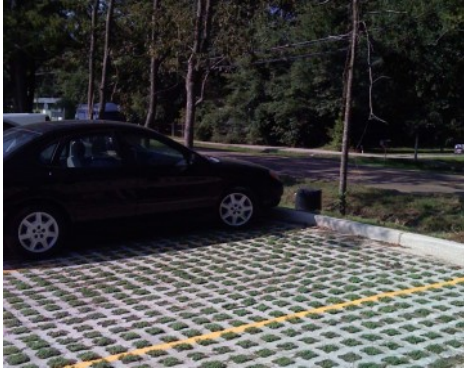
LA Army National Guard - Grasscrete Parking Lot
