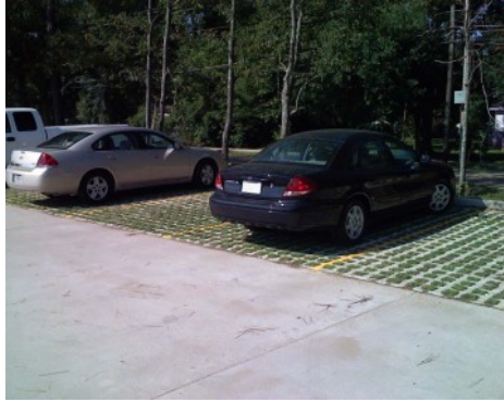
LA Army National Guard - Grasscrete Parking Lot
