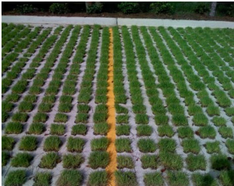
LA Army National Guard - Grasscrete Parking Lot
