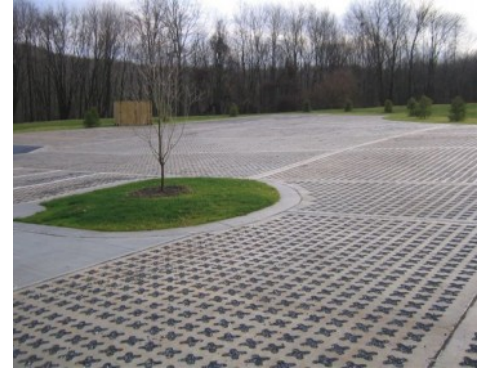
Plumway II Building Parking Lot - Stone Filled Grasscrete
