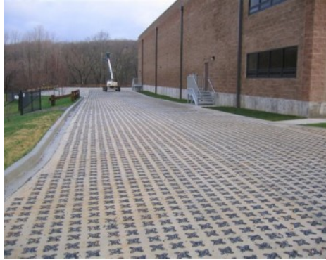
Plumway II Building Parking Lot - Stone Filled Grasscrete
