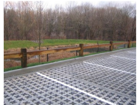
Plumway II Building Parking Lot - Stone Filled Grasscrete
