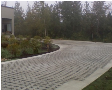
Micronics - Truck Dock Access - Stone Filled Grasscete
