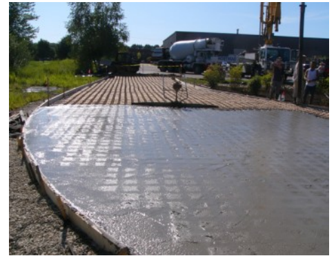
Micronics - Truck Dock Access - Stone Filled Grasscete
