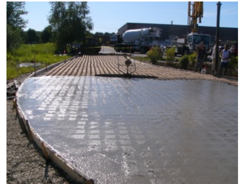
Micronics - Truck Dock Access - Stone Filled Grasscete
