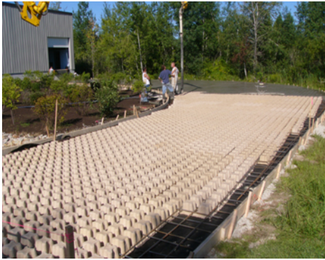
Micronics - Truck Dock Access - Stone Filled Grasscete
