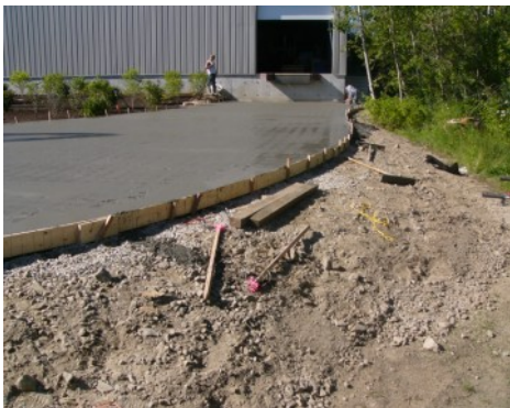
Micronics - Truck Dock Access - Stone Filled Grasscete
