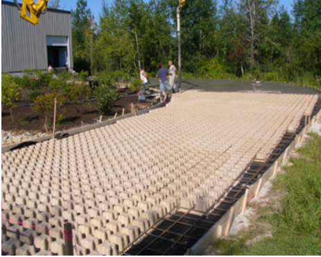
Micronics - Truck Dock Access - Stone Filled Grasscete
