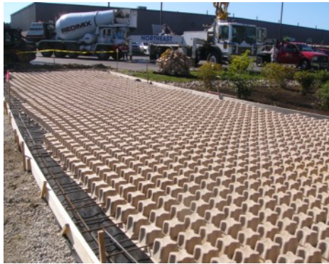
Micronics - Truck Dock Access - Stone Filled Grasscete
