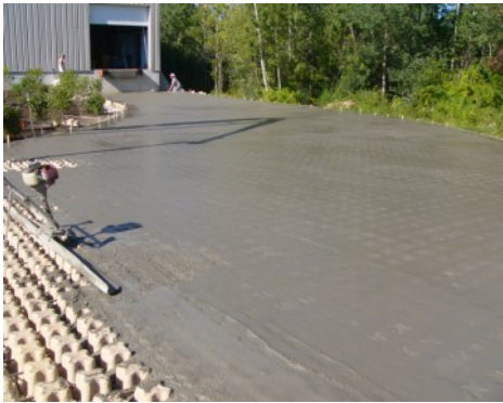
Micronics - Truck Dock Access - Stone Filled Grasscete
