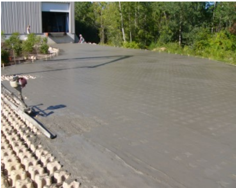
Micronics - Truck Dock Access - Stone Filled Grasscete
