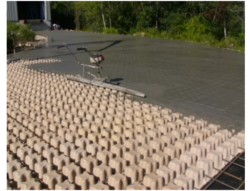
Micronics - Truck Dock Access - Stone Filled Grasscete
