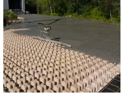
Micronics - Truck Dock Access - Stone Filled Grasscete
