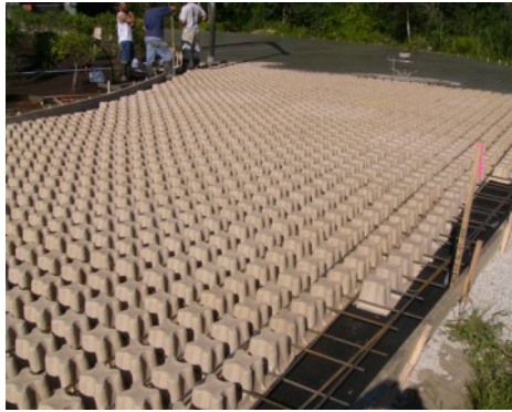
Micronics - Truck Dock Access - Stone Filled Grasscete
