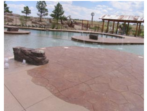
Idyllwilde Recreation Center - Mixed Use Bomanite Imprinted Concrete and Bomanite Sandstone Texture
