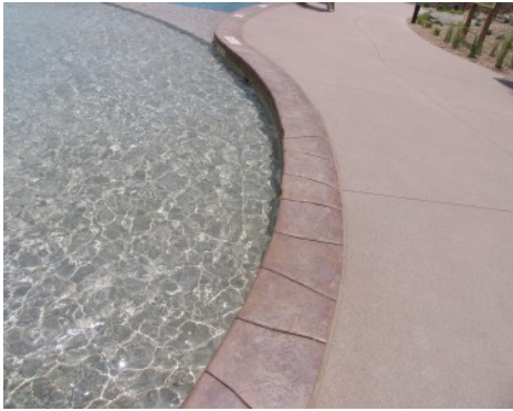
Idyllwilde Recreation Center - Mixed Use Bomanite Imprinted Concrete and Bomanite Sandstone Texture
