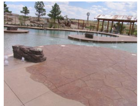
Idyllwilde Recreation Center - Mixed Use Bomanite Imprinted Concrete and Bomanite Sandstone Texture
