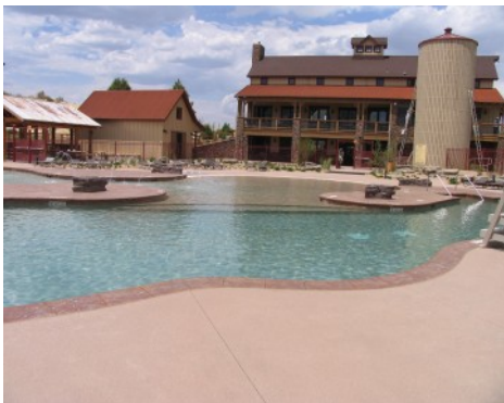
Idyllwilde Recreation Center - Mixed Use Bomanite Imprinted Concrete and Bomanite Sandstone Texture
