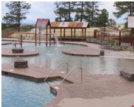
Idyllwilde Recreation Center - Mixed Use Bomanite Imprinted Concrete and Bomanite Sandstone Texture
