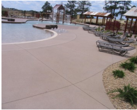
Idyllwilde Recreation Center - Mixed Use Bomanite Imprinted Concrete and Bomanite Sandstone Texture
