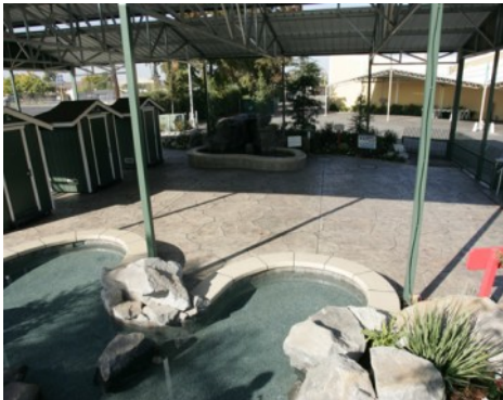
Fresno Fairgrounds Entrance - Bomanite Imprinted Concrete
