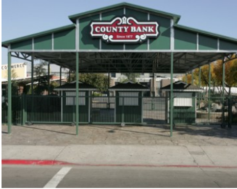
Fresno Fairgrounds Entrance - Bomanite Imprinted Concrete
