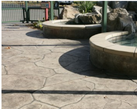
Fresno Fairgrounds Entrance - Bomanite Imprinted Concrete
