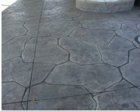
Fresno Fairgrounds Entrance - Bomanite Imprinted Concrete
