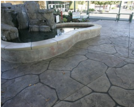
Fresno Fairgrounds Entrance - Bomanite Imprinted Concrete
