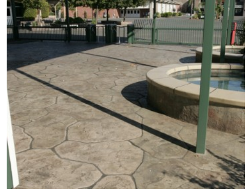
Fresno Fairgrounds Entrance - Bomanite Imprinted Concrete
