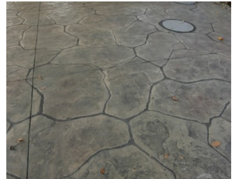
Fresno Fairgrounds Entrance - Bomanite Imprinted Concrete
