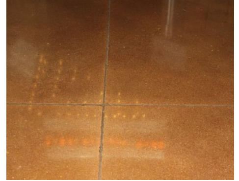
The Summit Recreation Center - Bomanite Integrally Colored Polished Concrete Floor - Close Up
