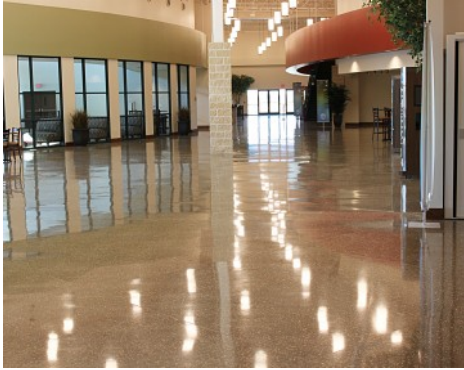
Prestonwood Baptist Church - Bomanite Custom Polished Concrete - Renaissance System
