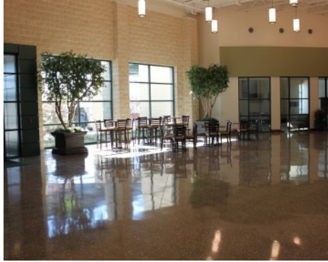
Prestonwood Baptist Church - Bomanite Custom Polished Concrete - Renaissance System
