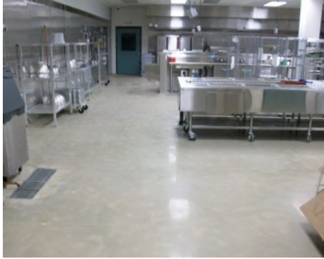
Cheshire County Jail Kitchen Floor - Bomanite Custom Polished Concrete Belcolore System
