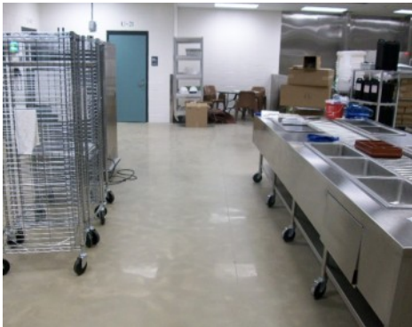
Cheshire County Jail Kitchen Floor - Bomanite Custom Polished Concrete Belcolore System
