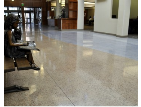
Loveland Library - Custom Polished Concrete - Bomanite Modena
