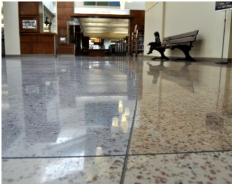
Loveland Library - Custom Polished Concrete - Bomanite Modena
