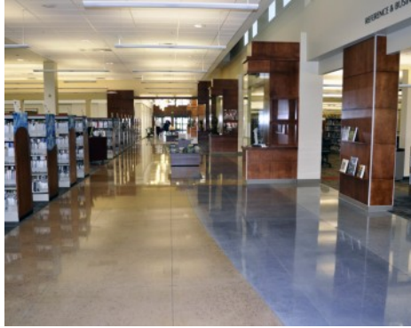
Loveland Library - Custom Polished Concrete - Bomanite Modena
