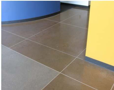
Fitzsimmons Educational Center - Bomanite Custom Polished Floor - Patene Teres Concrete Dye
