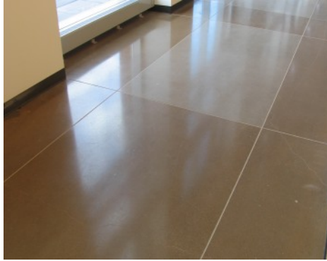
Fitzsimmons Educational Center - Bomanite Custom Polished Floor - Patene Teres Concrete Dye
