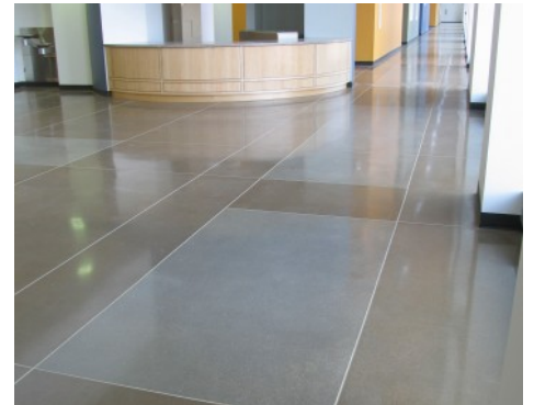
Fitzsimmons Educational Center - Bomanite Custom Polished Floor - Patene Teres Concrete Dye
