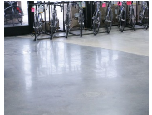
Tri-Sport Bicycle Shop - Custom Polished Concrete Floor - Integrally Colored with Imbeds
