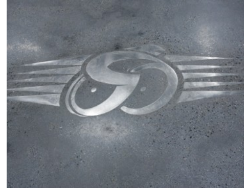
Tri-Sport Bicycle Shop - Custom Polished Concrete Floor - Integrally Colored with Imbeds
