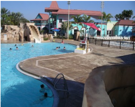
The Caribbean Beach Resort - Old Port Royal Swimming Pool - Bomanite Imprint Systems
