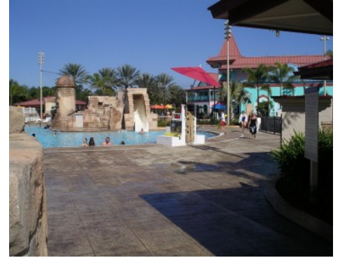
The Caribbean Beach Resort - Old Port Royal Swimming Pool - Bomanite Imprint Systems
