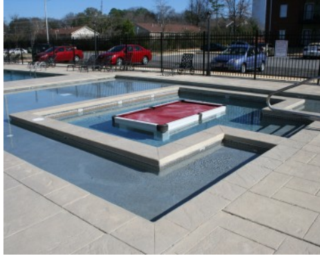
University Village Apartments Pool Deck - Bomanite Imprint Systems Large Ashlar Slate
