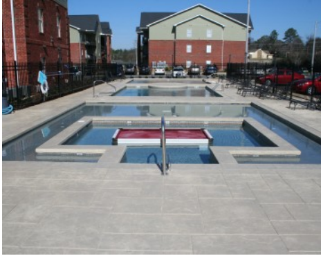
University Village Apartments Pool Deck - Bomanite Imprint Systems Large Ashlar Slate
