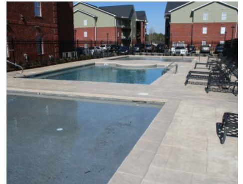
University Village Apartments Pool Deck - Bomanite Imprint Systems Large Ashlar Slate
