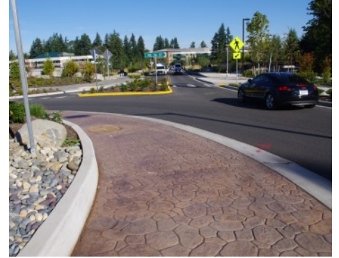
Washington NE 36th Street Bridge Roundabout - Bomanite Imprint Systems - Bomacron Creek Stone Pattern
