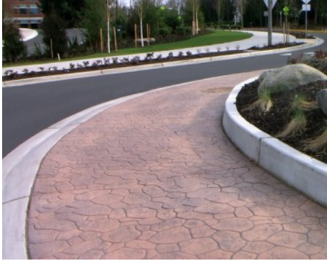
Washington NE 36th Street Bridge Roundabout - Bomanite Imprint Systems - Bomacron Creek Stone Pattern
