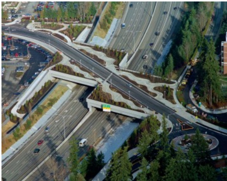
Washington NE 36th Street Bridge Roundabout - Bomanite Imprint Systems - Bomacron Creek Stone Pattern
