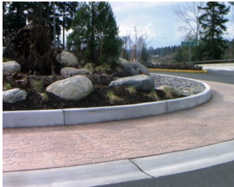
Washington NE 36th Street Bridge Roundabout - Bomanite Imprint Systems - Bomacron Creek Stone Pattern
