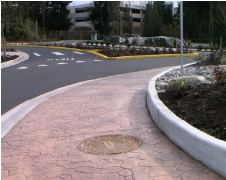
Washington NE 36th Street Bridge Roundabout - Bomanite Imprint Systems - Bomacron Creek Stone Pattern
