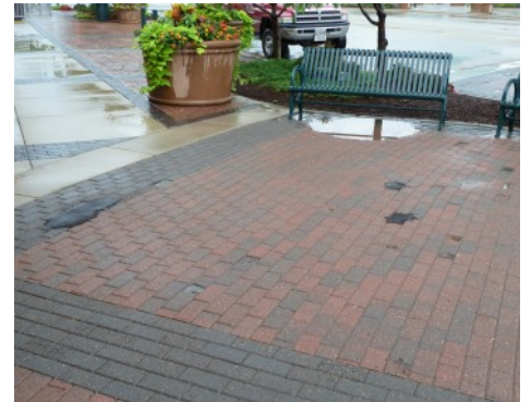
Greenway Station - Paver Replacement Before Image
