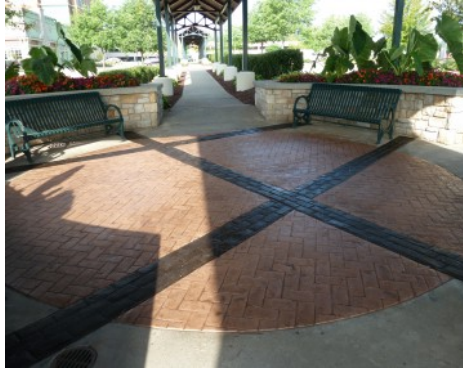
Greenway Station - Paver Replacement with Bomanite Imprint Systems
