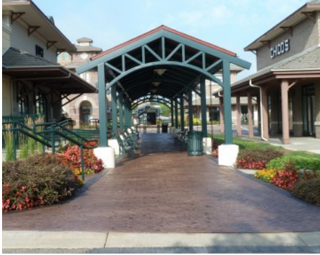
Greenway Station - Paver Replacement with Bomanite Imprint Systems
