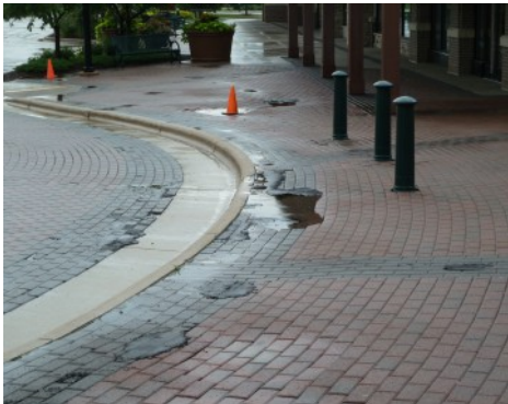
Greenway Station - Paver Replacement Before Image
