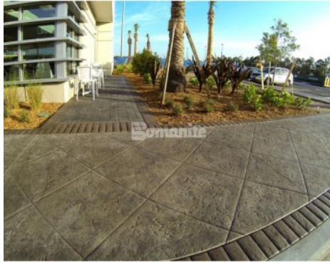
Florida Turnpike Ft Drum - Bomanite Imprint Systems; Coquina Texture, Soldier Course Brick, 6 x 6 Granite Setts
