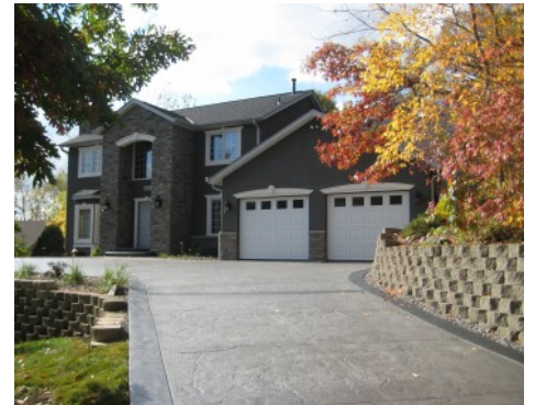
Bomanite Imprinted Concrete Driveway - Slate Texture
