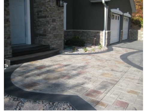
Bomanite Imprinted Concrete Front Entrance - Ashlar Slate Pattern
