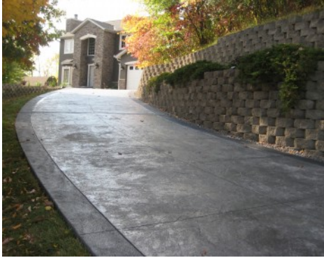
Bomanite Imprinted Concrete Driveway - Slate Texture
