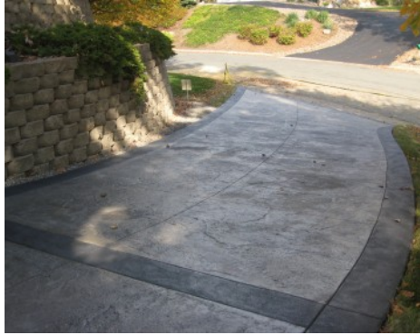
Bomanite Imprinted Concrete Driveway - Slate Texture
