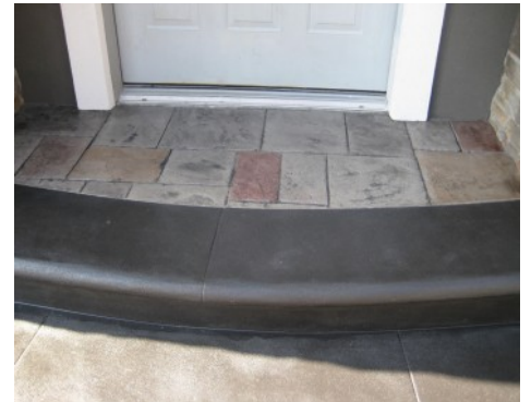
Bomanite Imprinted Concrete Front Entrance - Ashlar Slate Pattern
