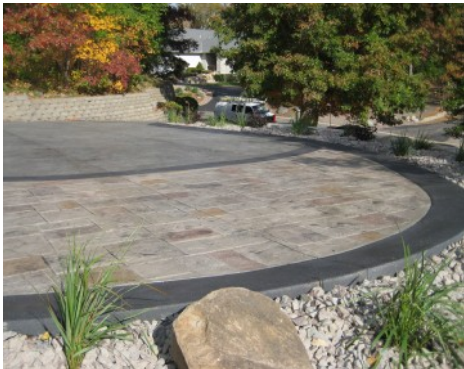
Bomanite Imprinted Concrete Driveway - Slate Texture with Ashlar Slate Pattern
