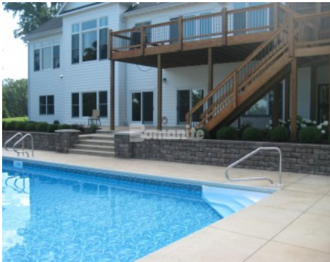
Residential Pool Deck - Bomanite Slate Texture
