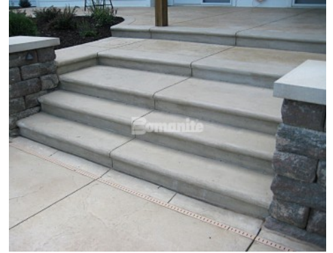
Residential Pool Deck Stairs - Bomanite Slate Texture
