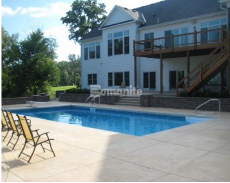
Residential Pool Deck - Bomanite Slate Texture
