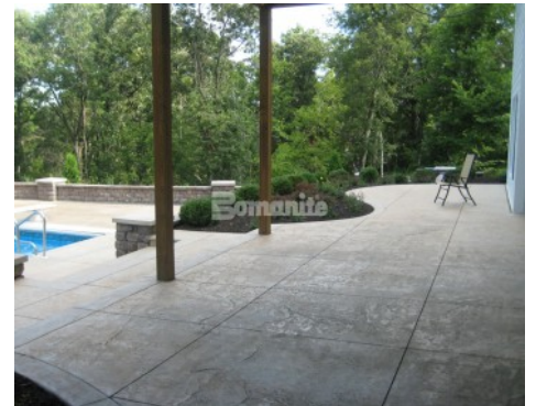
Residential Patio and Pool Deck - Bomanite Slate Texture
