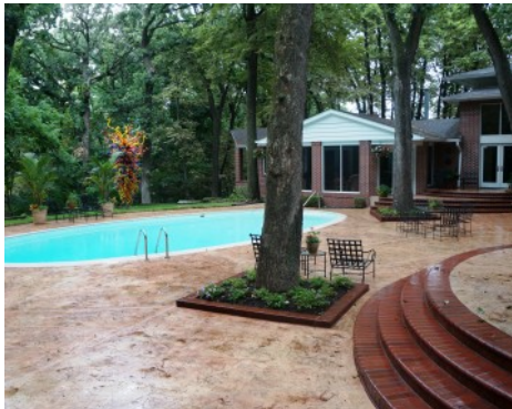
Residential Patio and Pool Deck - Bomanite Imprint Systems - Slate Texture
