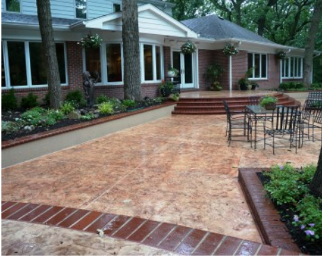
Patio and Pool Deck - Bomanite Imprint Systems - Slate Texture and Soldier Course Used Brick Border
