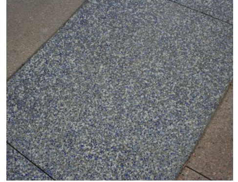
Centennial Center Park - Bomanite Revealed Close Up
