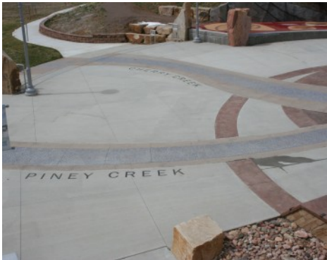
Centennial Center Park - Bomanite Sandstone Texture. Bomanite Revealed and Bomanite Imprint Systems Plaza
