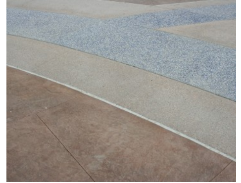
Centennial Center Park - Bomanite Sandstone Texture. Bomanite Revealed and Bomanite Imprint Systems
