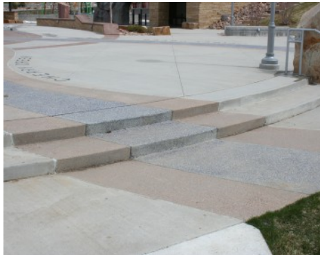
Centennial Center Park - Bomanite Sandstone Texture, Bomanite Revealed and Bomanite Imprint Systems Plaza
