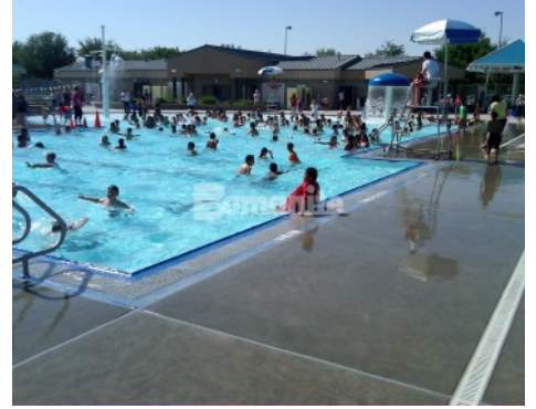
Central East High School Fresno - Bomanite Sandstone Texture Exposed Aggregate Pool Deck
