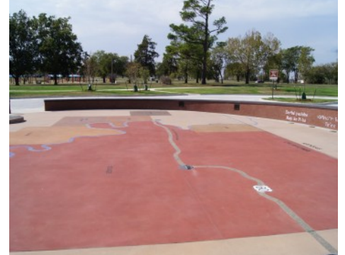
Standing Bear Museum - Exposed Aggregate Systems Bomanite Revealed and Bomanite Sandstone
