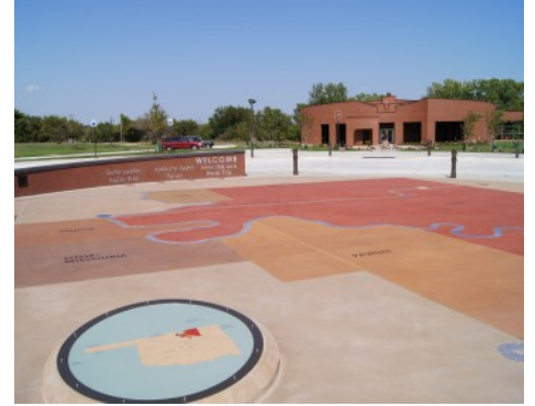
Standing Bear Museum - Exposed Aggregate Systems Bomanite Revealed and Bomanite Sandstone
