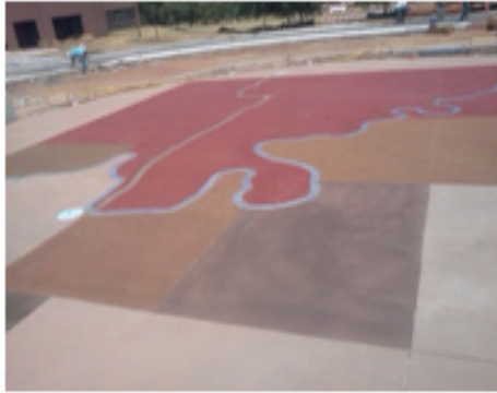
Standing Bear Museum - Exposed Aggregate Systems Bomanite Revealed and Bomanite Sandscape
