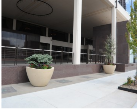
Marriott Hotel Downtown Kansas City - Bomanite Sandscape and Revealed
