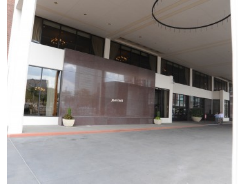
Marriott Hotel Downtown Kansas City - Bomanite Sandscape and Revealed
