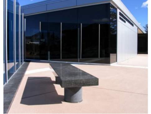
Asian Memorial - Bomanite Sandstone Texture Exterior Walk, Polished Concrete Bench
