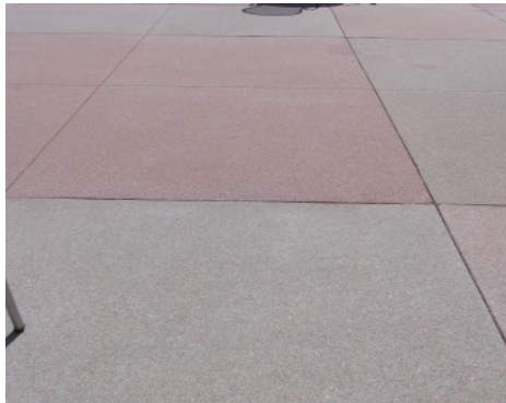
NCSL Building Plaza - Bomanite Sandscape Texture
