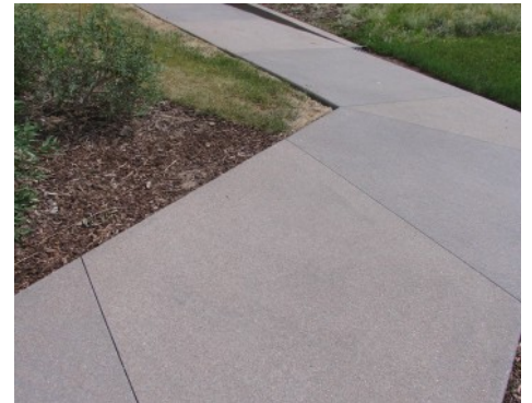
Powehouse Plaza - Bomanite Sandscape Texture
