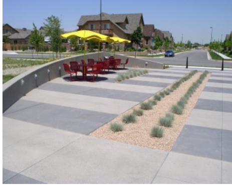
Powehouse Plaza - Bomanite Sandscape Texture
