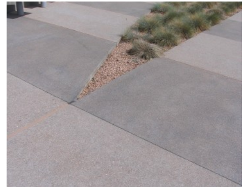
Powehouse Plaza - Bomanite Sandscape Texture
