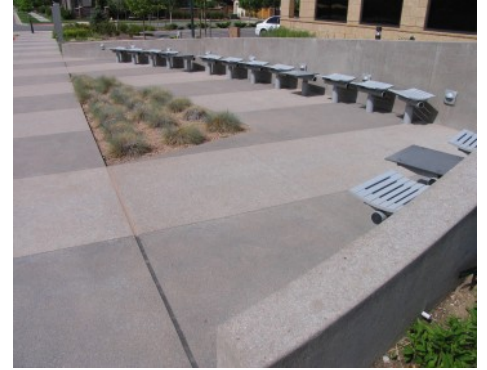
Powehouse Plaza - Bomanite Sandscape Texture
