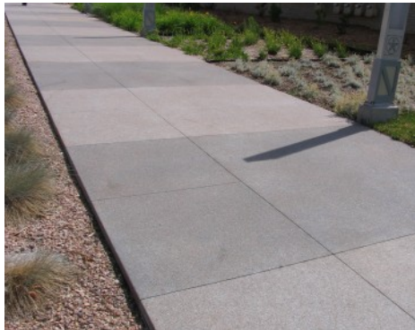
Powehouse Plaza - Bomanite Sandscape Texture
