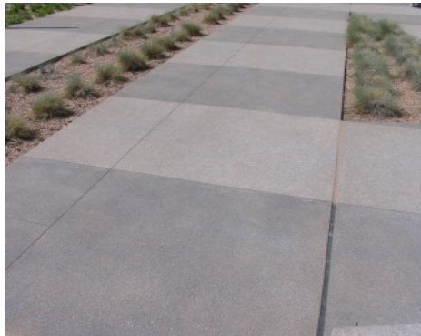
Powehouse Plaza - Bomanite Sandscape Texture
