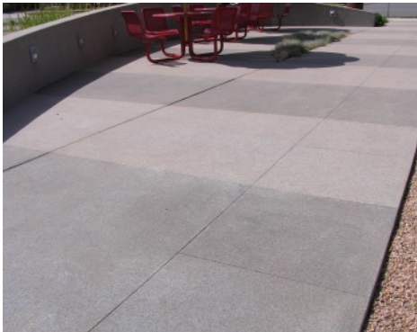
Powehouse Plaza - Bomanite Sandscape Texture
