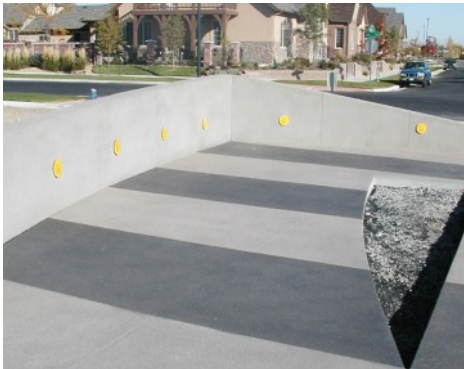
Powehouse Plaza - Bomanite Sandscape Texture
