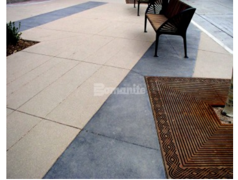
Stapleton Town Center Redevelopment - Bomanite Sandscape Texture Exposed Aggregate System
