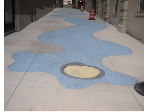
The Commons Baltimore Alley - Bomanite Revealed
