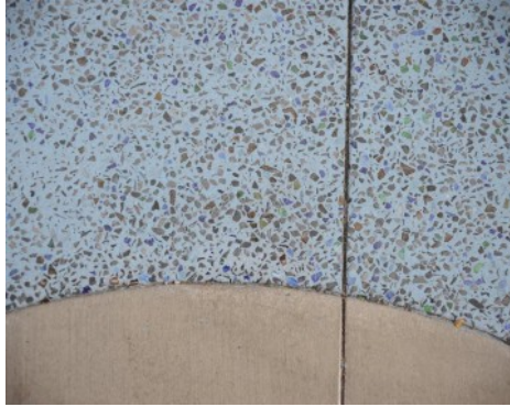
The Commons Baltimore Alley - Bomanite Revealed Close Up
