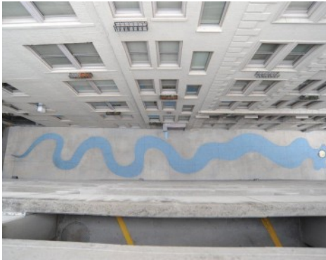
The Commons Baltimore Alley - Bomanite Revealed View from Above
