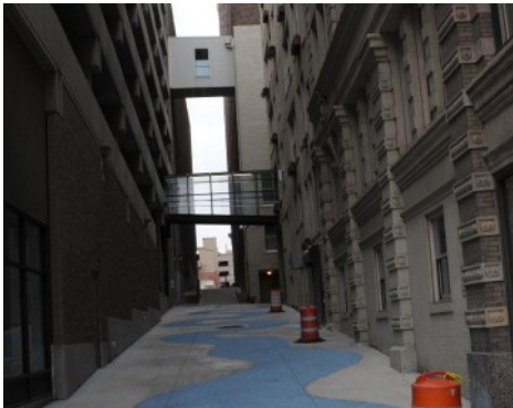
The Commons Baltimore Alley - Bomanite Revealed
