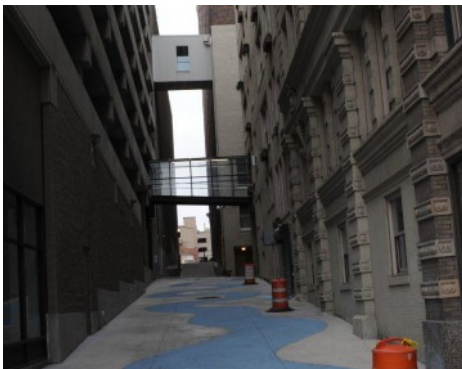
The Commons Baltimore Alley - Bomanite Revealed
