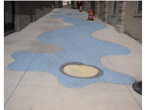
The Commons Baltimore Alley - Bomanite Revealed
