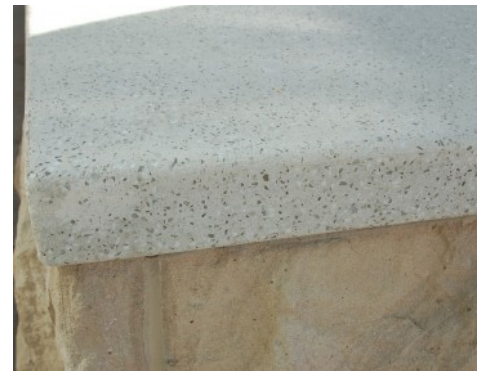
The Spire Pool Deck - Close Up - Bomanite Revealed Exposed Aggregate
