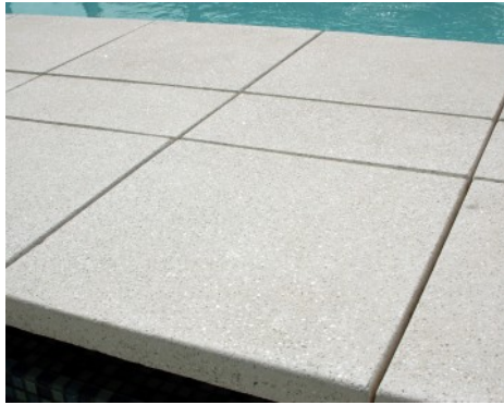
The Spire Pool Deck - Close Up - Bomanite Revealed Exposed Aggregate
