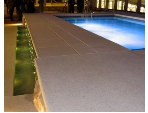
The Spire Pool Deck - At Night - Bomanite Revealed Exposed Aggregate
