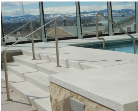
The Spire Pool Deck - Bomanite Revealed Exposed Aggregate
