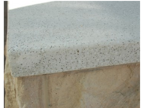
The Spire Pool Deck - Close Up - Bomanite Revealed Exposed Aggregate
