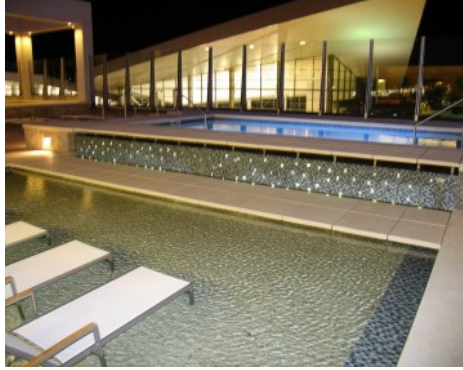
The Spire Pool Deck - At Night - Bomanite Revealed Exposed Aggregate
